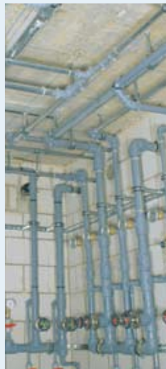
Hot and cold water in INS
