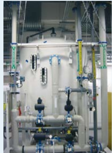
DI water/specified water in PROGEF® Plus.
